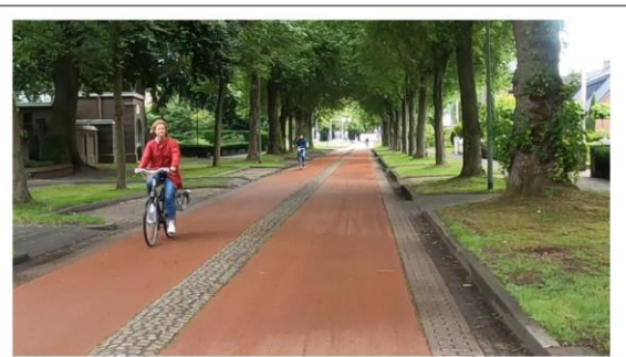
A cycle street in Oss. The strips on the far side of the street act as rumble strips and optically narrow this cycle street. The central strip is slightly raised to also act as a rumble strip and to force drivers to overtake at a safe distance (completely in the opposite lane).
