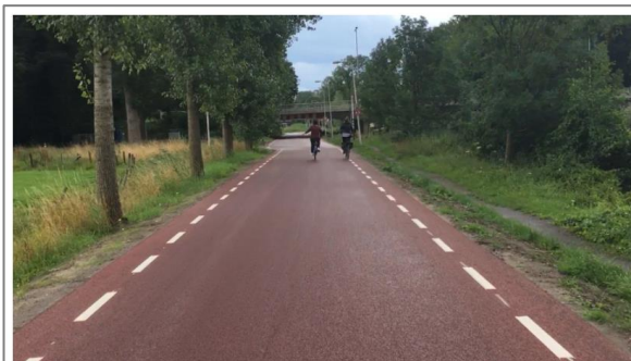
Advisory lanes done right. There is no confusion here as to what they are. Merely lines to optically narrow the road (a cycle street in this case, that is why the asphalt is red) to get the speed of motor traffic down.
